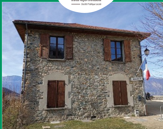
Energy renovation project at Venon town hall
