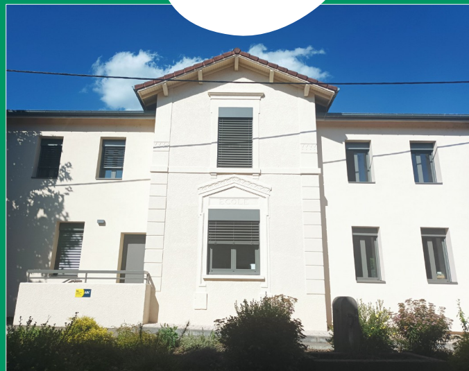
Renovation of Ambutrix primary school
