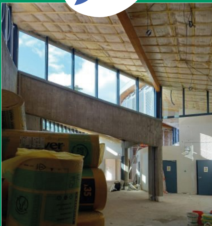
Renovation project at Vourles school (69)
